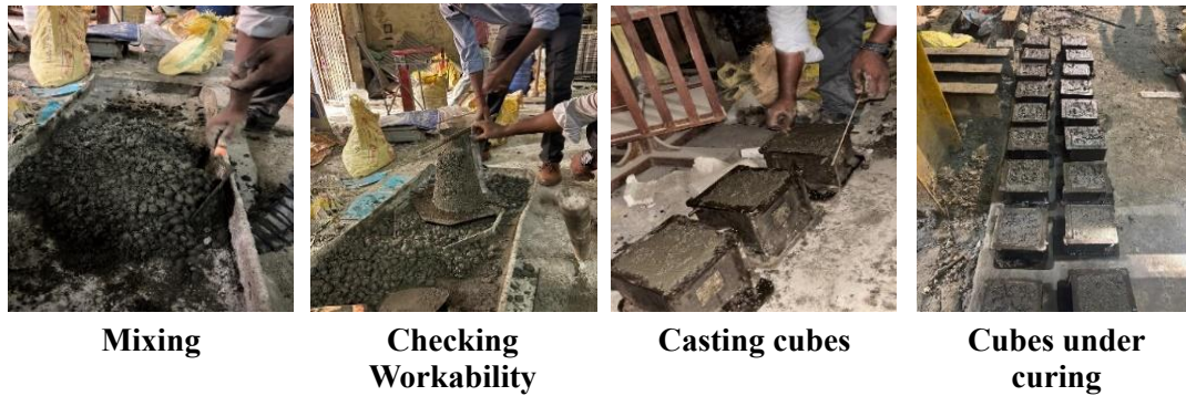
Fig 2. Cube casting and curing
