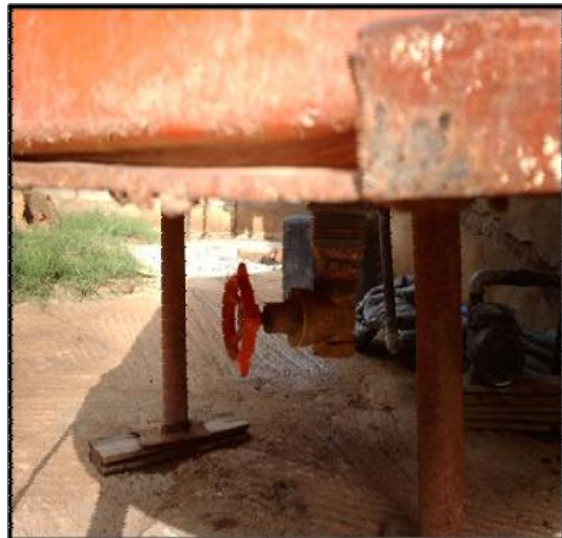
Plate 4: Tank Support with Valve
