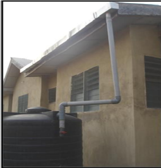
Plate 1: Tank with Pipe
